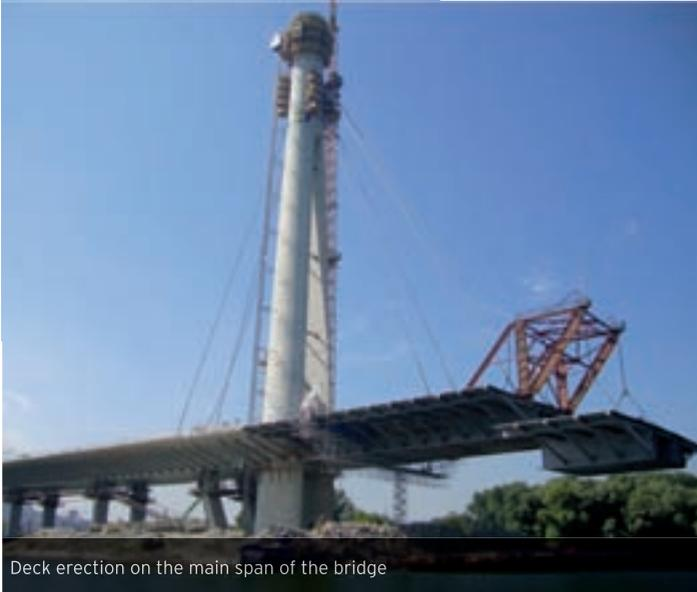
Deck erection on the main span of the bridge
