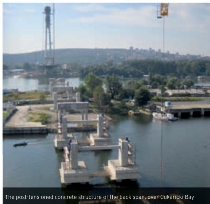
The post-tensioned concrete structure of the back span, over Cukaricki Bay
