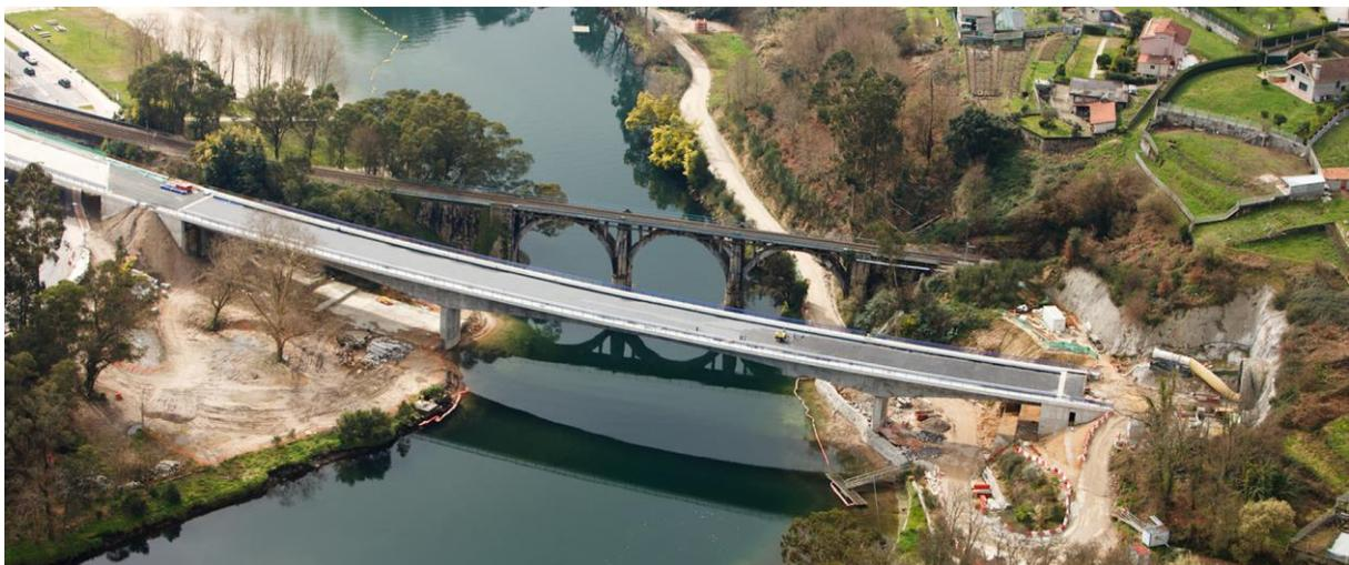
The 171-meter-long, 3-span San Benito viaduct over the Lerez River is a high speed railway bridge near the city of Pontevedra in northwest Spain. The superstructure is a single cell box post-tensioned haunch
