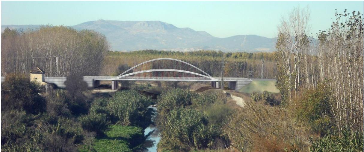
Louis Berger designed the viaduct over the Genil River, a highway bridge located at the Granada External Bypass in the south of Spain. The three-span, 110-meter-long bridge spans the river with an 80-meter-long tied arch. The 41.2-meter-wide superstructure includes three reinforced concrete arches – a central vertical arch and inclined arches on each side.
