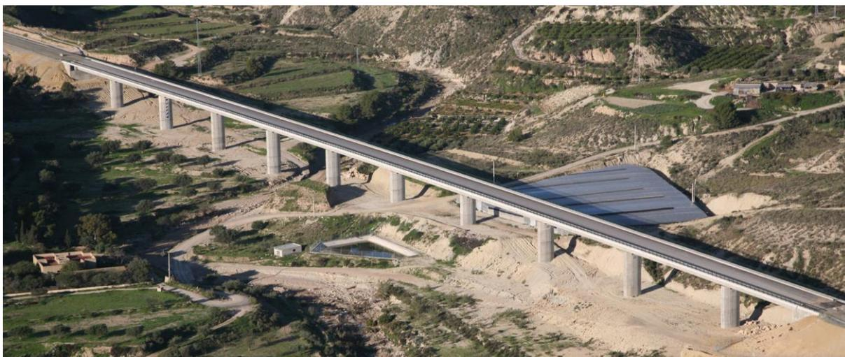
Three viaducts designed by Louis Berger have been built by means of a self-launching formwork gantry in the Los Gallardos – Sorbas segment of the high speed railway between Murcia and Almería in the southeast of Spain:
