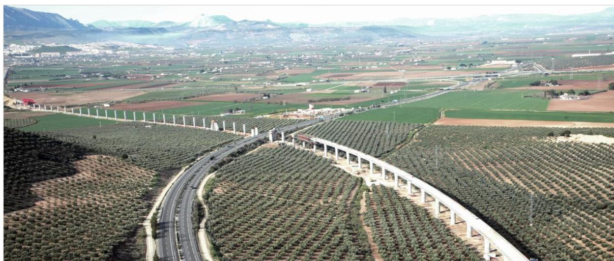
The Guadalhorce viaduct, designed by Louis Berger, is part of the high-speed rail line Antequera-Peña de los Enamorados in southern Spain. It stretches over 2,525 meters in length and consists of 49 spans, each 51.25 meters long. Situated in a medium-risk seismic zone, it is one of the longest bridges of its type in the country.
